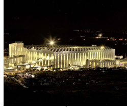
Saucito II commissioning
