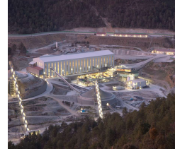
San Julián phase II commissioning
