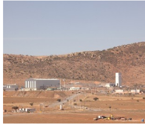
Saucito I commissioning
