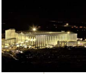
Saucito II commissioning
