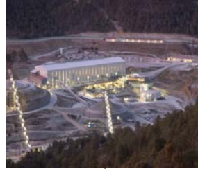
San Julián phase II commissioning
