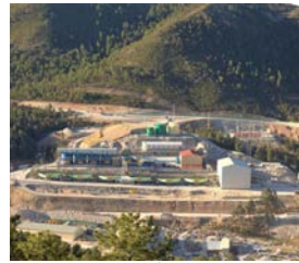
San Julián phase I commissioning
