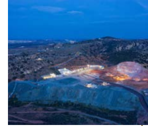
Juanicipio project construction completed in 4Q21
